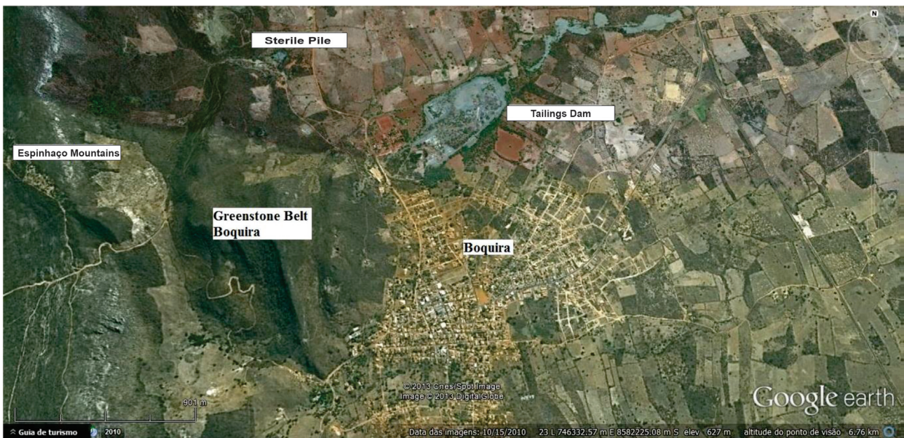
Figure 2: Disposal of tailings basin in the urban perimeter of the city of Boquira.
